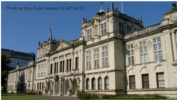
The Main Building, Cardiff University
